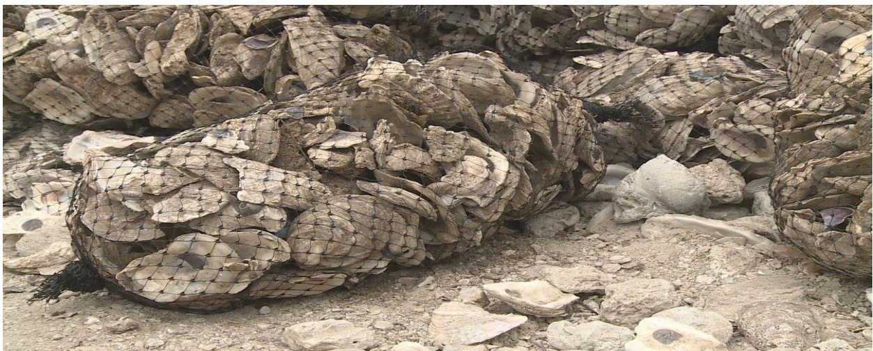
Slika 14. Grebeni od ljuštura kamenica u polietilenskim vrećama. ( https://www.wjhg.com/content/news/Oyster-shell-reefs-help-restore-Choctawhatchee-shoreline-425406014.html )
