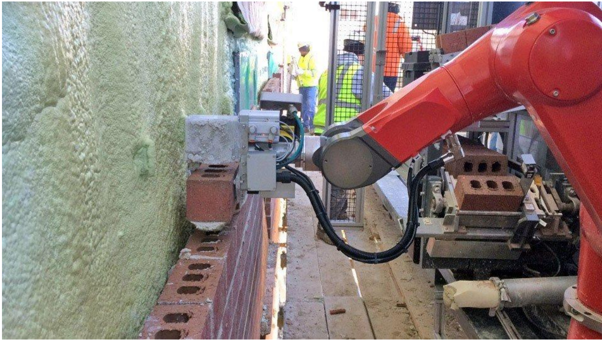
Slika 8. SAM (izvor: https://www.techexplorist.com/meet-sam-construction-robot-works-500-faster-humans/5357/ )
