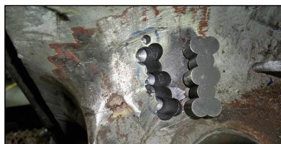
Izvor: QuantiServ, dostupno na: <https://www.quantiserv.com/solutions/metal-stitching/>
