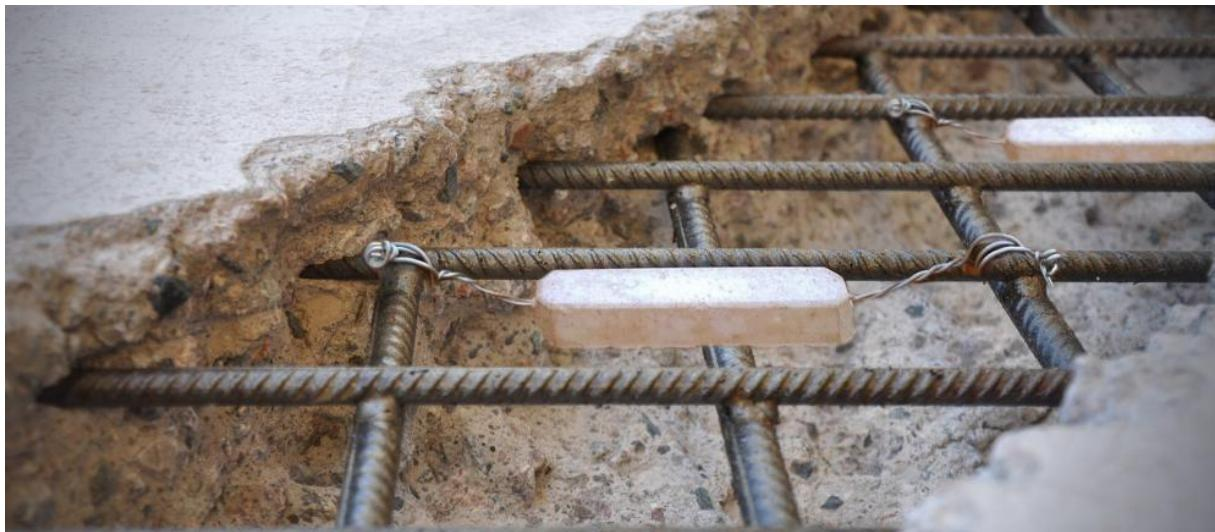
Slika 15 Primjer pasivne katodne zaštite na armaturi armiranog betona. Izvor: [https://www.vector-corrosion.com/uploads/content/fullsize/water\\_jet\\_power1.jpg](https://www.vector-corrosion.com/uploads/content/fullsize/water_jet_power1.jpg)
