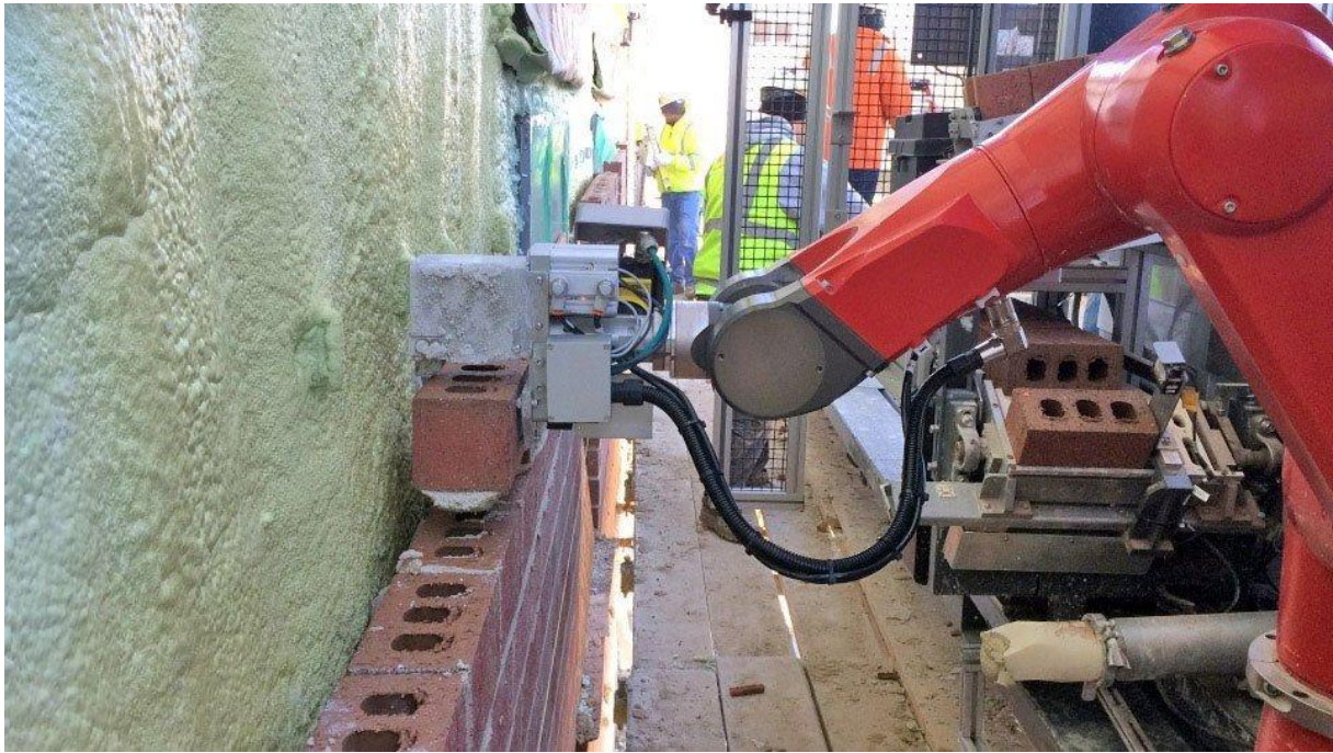
Slika 8. SAM (izvor: https://www.techexplorist.com/meet-sam-construction-robot-works-500-faster-humans/5357/ )
